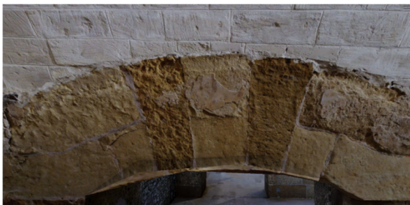
Figure 18: Erosion in the limestone: displaying Matterport model on Unity Platform.
