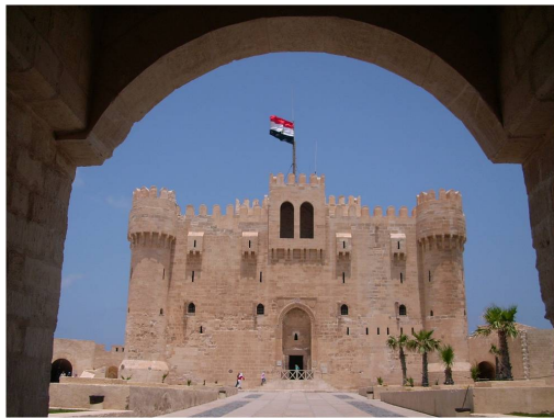
Figure 4: The main standalone tower
