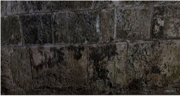
Figure 20: Capillarity in the limestone of the coastal passage: Matterport model on Unity Platform.
