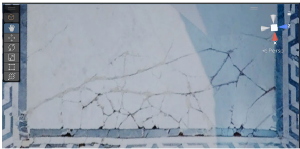
Figure 17: Visible cracks in the precious marble floor of the Vestibule Matterport model on Unity Platform.
