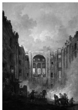
Figure 6. Interior of the Opera House of the Palais Royal the Day after the Fire (Dubin, 2012: 63).
